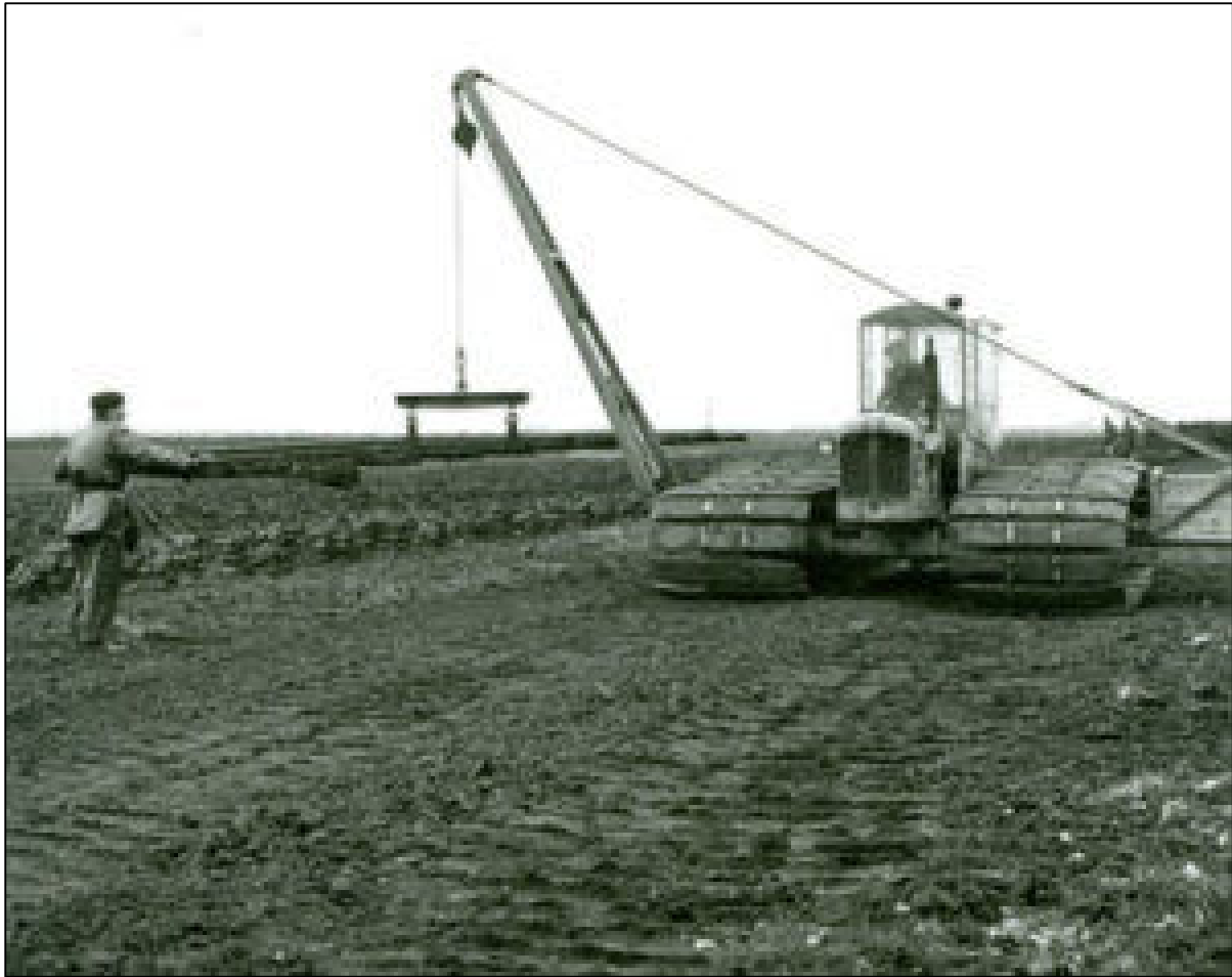
Plate 4-41: Rail Moving Attachment to lift and lay temporary railway track, along sod peat ricks and milled peat piles. (source: https://www.bordnamonalivinghistory.ie/equipment-detail/rail-moving-attachment/ )
