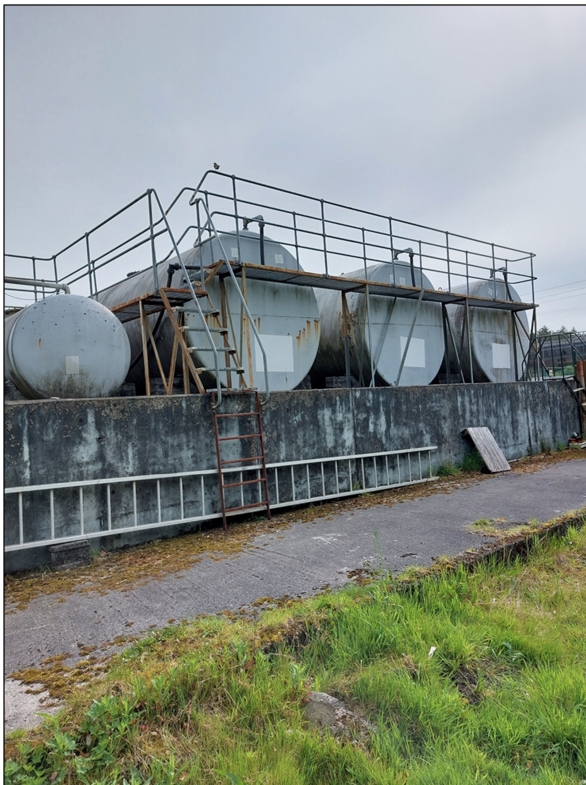
Plate 4-35: Existing fuel storage tanks with bunding at Mountdillon Works
